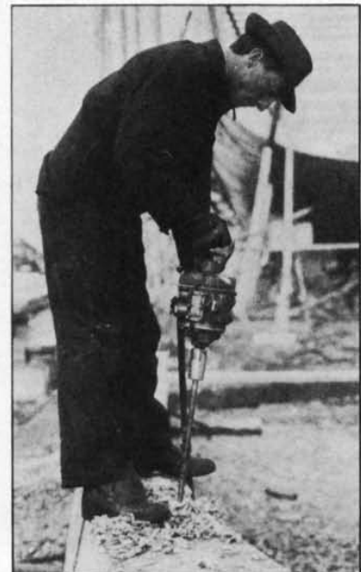
FIG. 11—BORING HOLES WITH AN AIR DRILL
