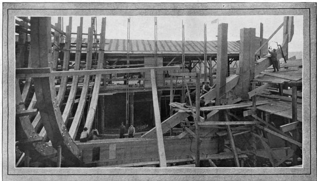
FIG. 105—ERECTING FORE AND AFT POST TIMBERS FOR A STERN OF UNUSUALLY STRONG CONSTRUCTION
