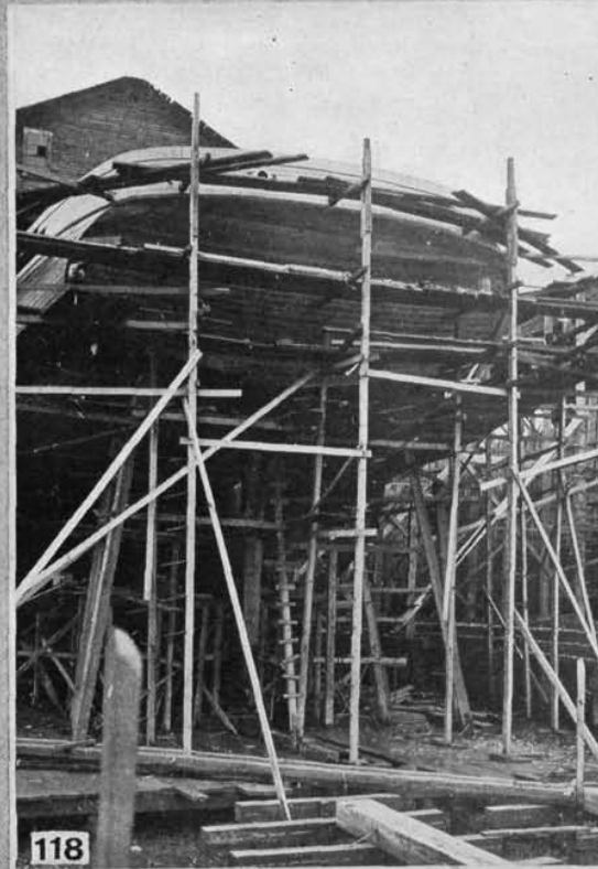
FIG. 115—DETAIL OF STERN FRAMING FROM THE INSIDE OF A SHIP. FIG. 116—ANOTHER VIEW OF THE FRAMING OF THE SAME SHIP. FIG. 117—LOWER PART OF STERN FRAMING OF THE SAME SHIP SHOWING STERN-POST, DEADWOOD, ETC. FIG. 118—SAME STERN PLANKED UP AND NEARLY FINISHED
