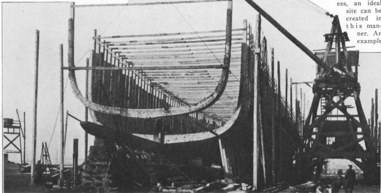
FIG. 16—ELECTRICALLY-DRIVEN, TRAVELING DERRICK SETTING FRAMES IN A WOODEN SHIPYARD
