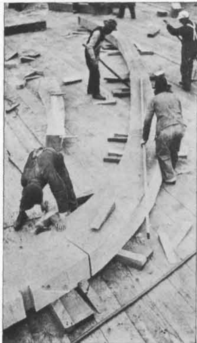
FIG. 51—ASSEMBLING FRAME FUTTOCKS ON FRAMING STAGE
