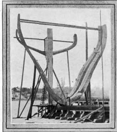
FIG. 100—DETAIL OF STERN FRAME OF SHIP BEING BUILT FOR UNITED STATES GOVERNMENT
