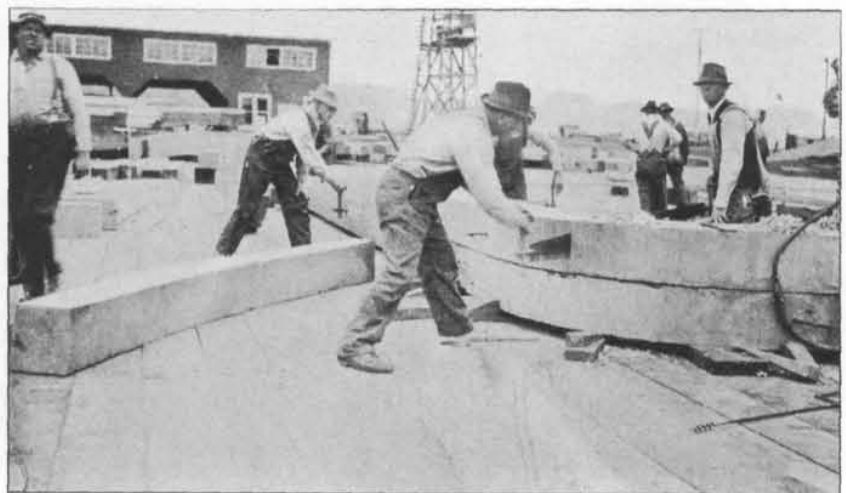
FIG. 52—RESAWING FRAME JOINTS TO A PROPER FIT
