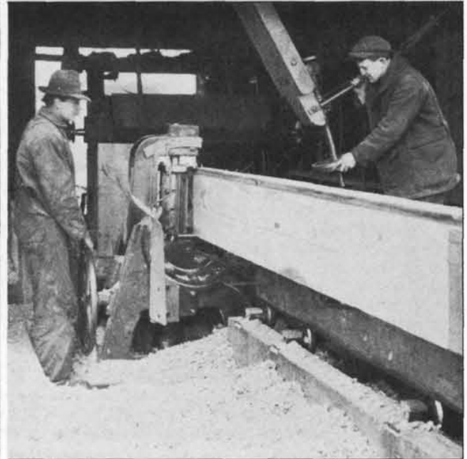
FIG. 9—SPECIAL MACHINES HAVE BEEN DESIGNED FOR BEVELING AND EDGING TIMBERS
